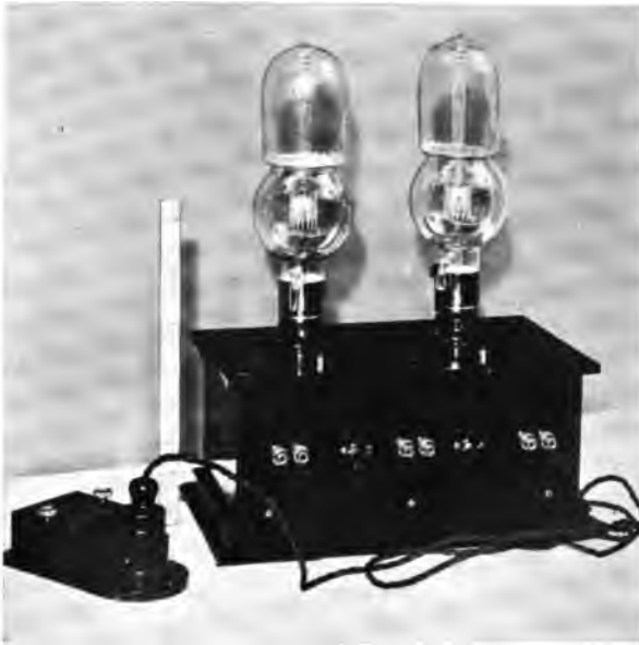
FIG. 79 a.—Lieben valves for intensification of spark signals.
